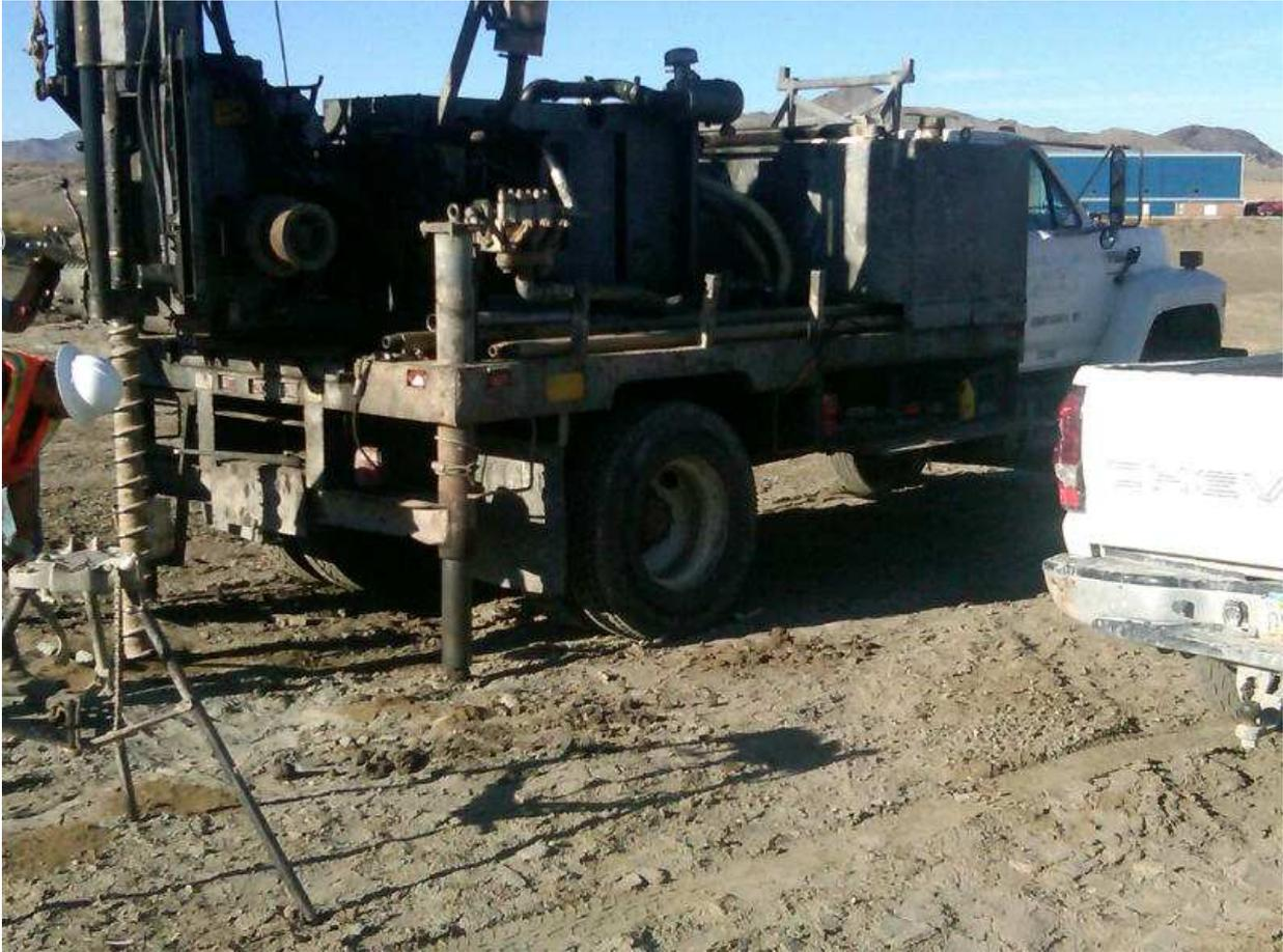
**Figure 1: Auger drilling on site**
